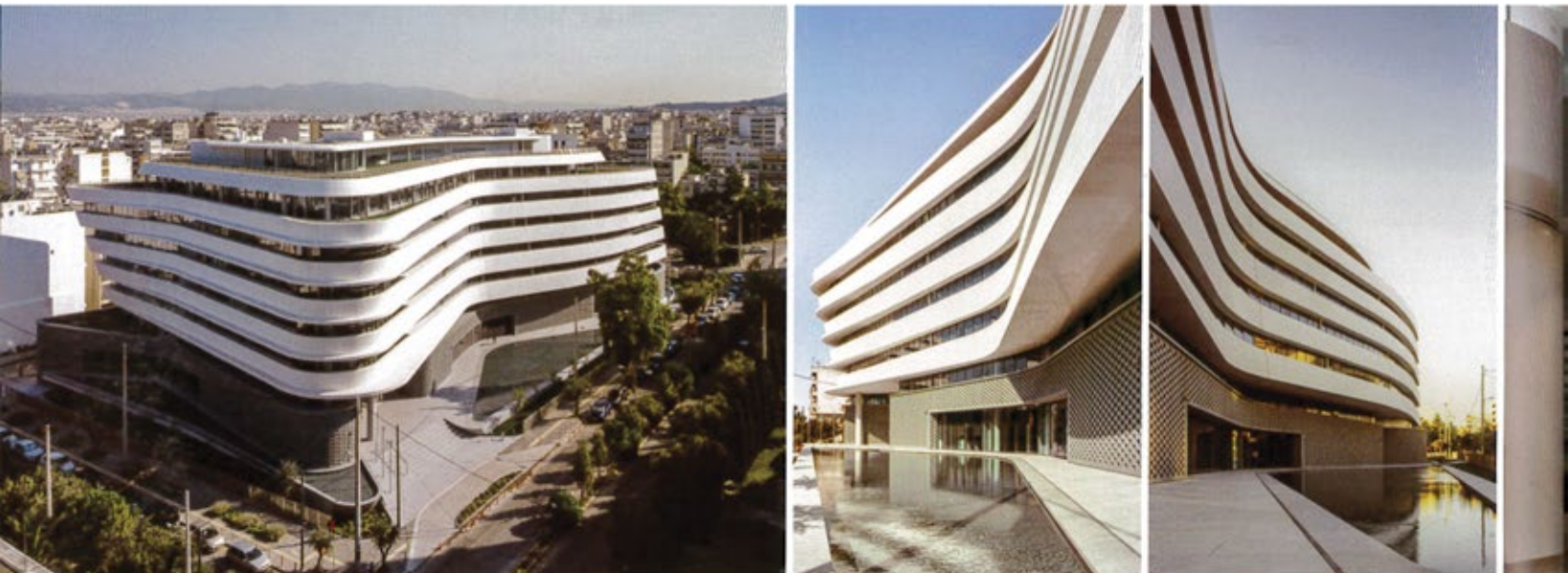
The ground floor of the headquarters features a perforated facade made of glass-fibre reinforced concrete and the upper floors have a white marble facade.
